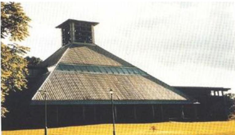
Photo 1: Wind tower ventilation
